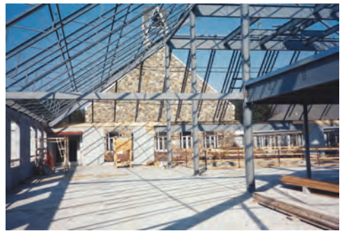
Phase II - the two-story Christian Education building under construction
