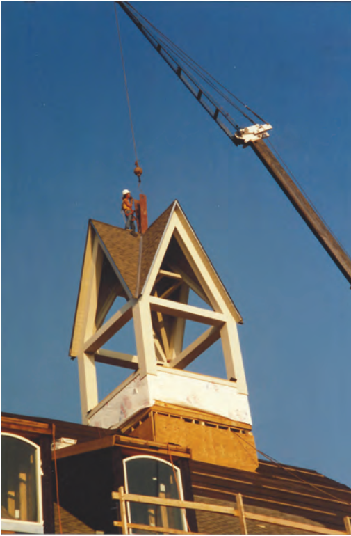
Placing the steeple, 1993
